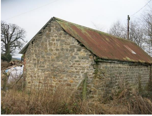
Photo 13 Stonework with crevices Building 3
