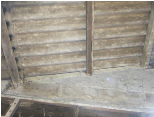
Photo 9 Asbestos with gap to wall top Building 2
