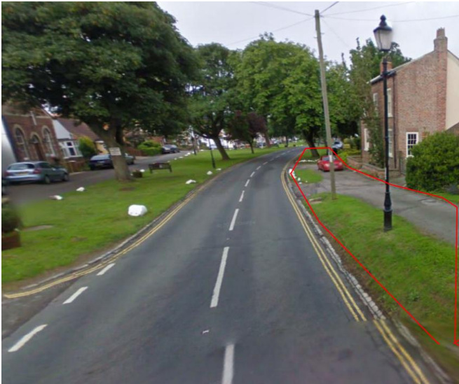
Figure 3 Potential Infrastructure Clashes with Elwick Road
