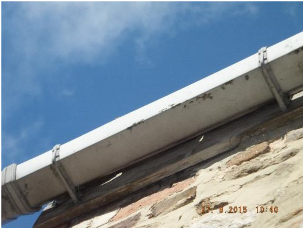
Photograph 18 Potential bat access point, Building C gap under fascia board
